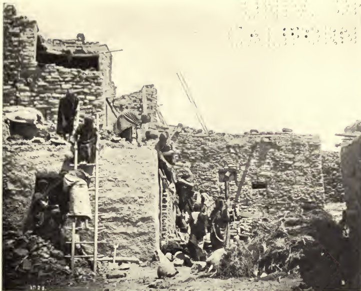
HOPI WOMEN BUILDING A HOUSE AT ORAIBI.
