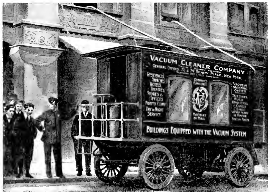
PORTABLE PLANT OF THE VACUUM CLEANER CO.
