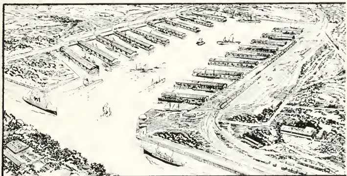
DOCKS AT COLON—PACIFIC TERMINUS, PANAMA CANAL
