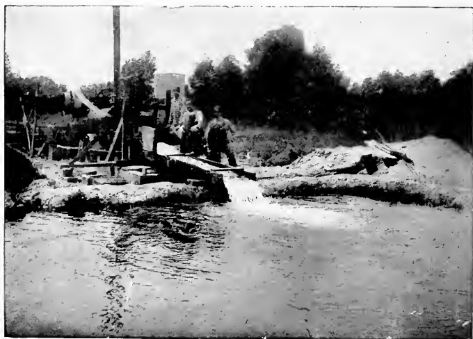
RICE PUMP IN ACTION AND IMPROVISED RESERVOIR
