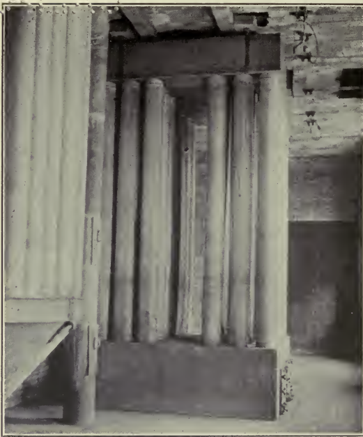
DUST COLLECTORS IN A LEAD PLANT
