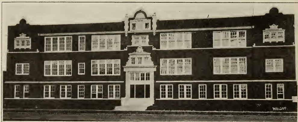
FIG. 2. FRONT OF VOCATIONAL BUILDING.
