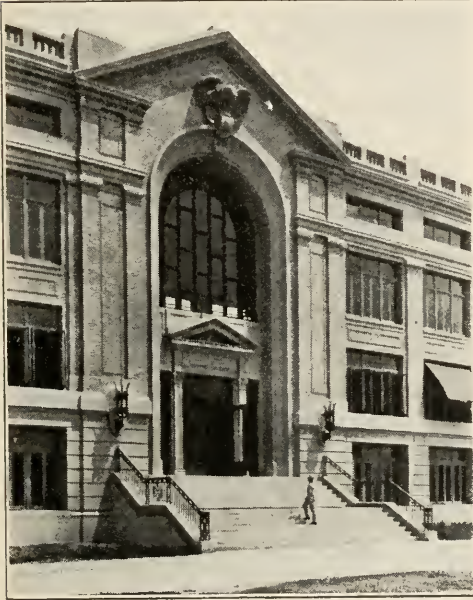
MAIN ENTRANCE, DELGARDO TRADE SCHOOL, NEW ORLEANS.
