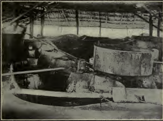
Fig. 34.—Open Pan Evaporators, Philippines. (Courtesy of the School of Mines Quarterly, Columbia University.)
