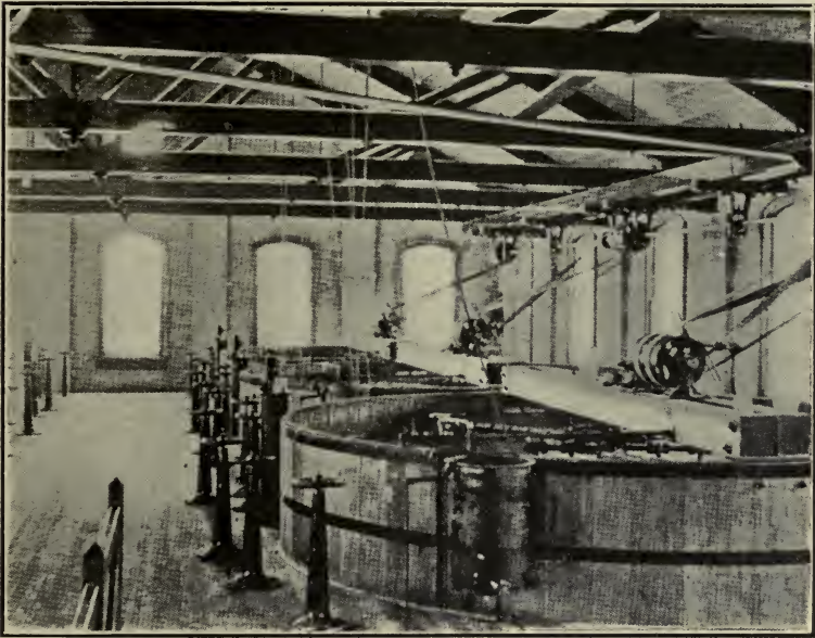
Fig. 4.—View of the Interior of the East Albany, N. Y., Filter-plant. (Courtesy of John Wiley & Sons.)
