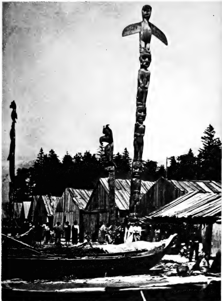
7. A Southern Kwakiutl village of the 1880s. The vertical planking on the houses is one effect of the availability of iron nails. The boldly simplified carvings are typical of Kwakiutl art prior to the influence of northern "totem pole" art.
