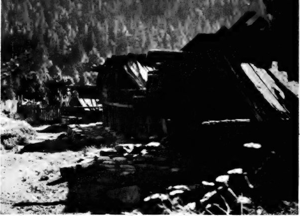
8. Yurok houses of redwood planks. Note the double slope of the roofs on the far side of both houses, which, with the slope nearest the camera, formed the typical "three-pitch" roof of the lower Klamath. A. L. Kroeber photograph.
