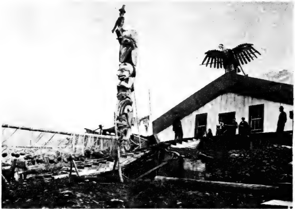
9. A chief's house in a Bella Coola village (probably Kimsquit), near the turn of the twentieth century. The house combines alien influences: the framed doorway and windows are of European source; the false plates and nailed vertical planking are imitations of aboriginal custom. Note the difference in the rather ponderous carving of the crest-display pole as compared to the vigorous old-style Kwakiutl carving and as well to the more stylized carving of the north. The gill net drying on the racks in the left foreground is a type of European commercial fishing net. Courtesy of the Smithsonian Institution.
