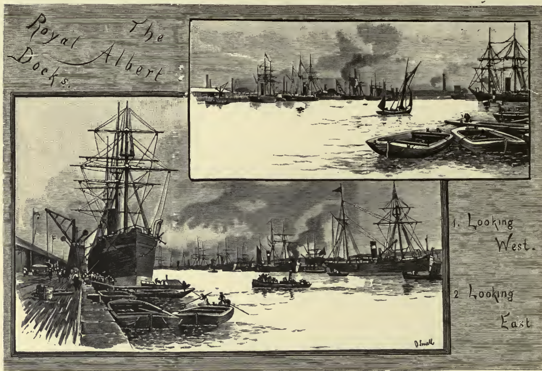
INSIDE THE BIG DOCKS.
