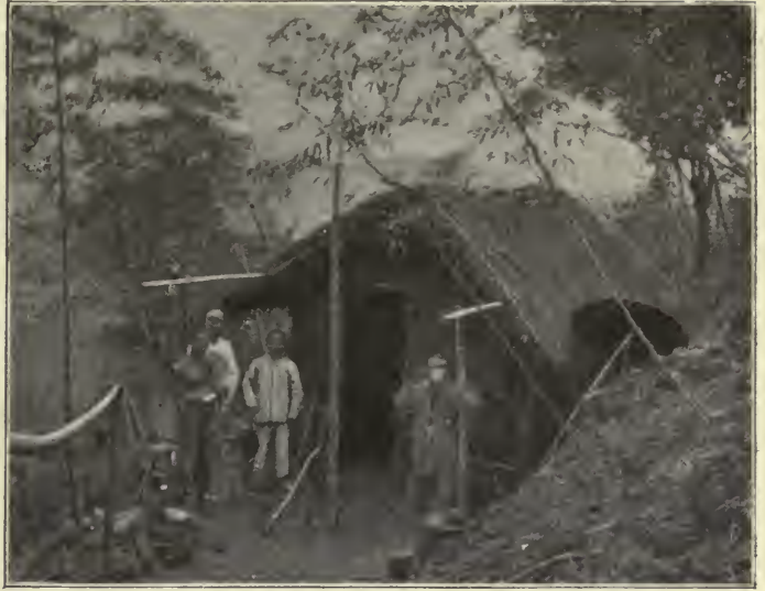
A WORKMAN'S HUT.
