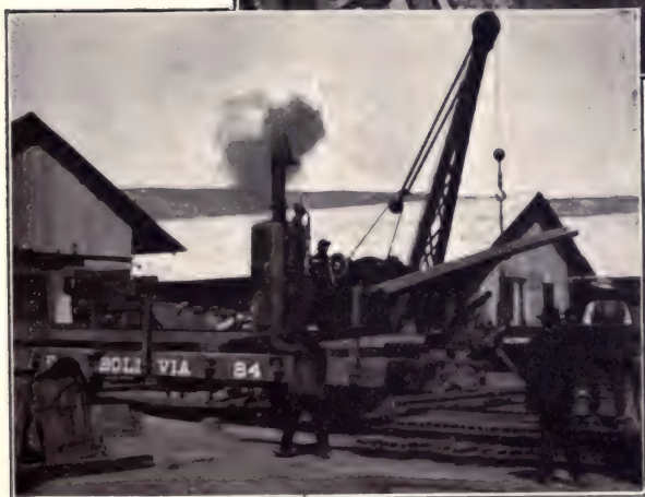
CONSTRUCTION WORK ON THE GUAQUI RAILROAD
