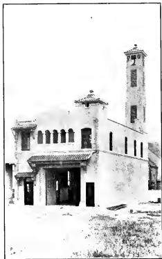
FIRE HOUSE, DEPT. NO. 1.
