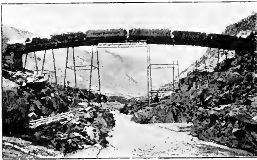
BRIDGE SEVENTY-FIVE FEET ABOVE LOWER TRACK.
