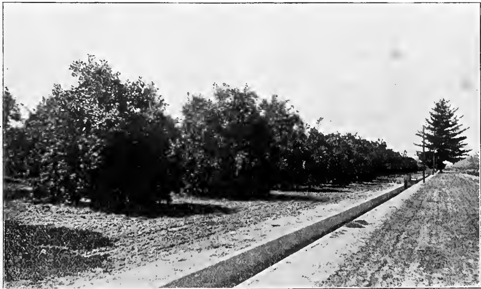
A CEMENTED IRRIGATION CANAL IN CALIFORNIA.
