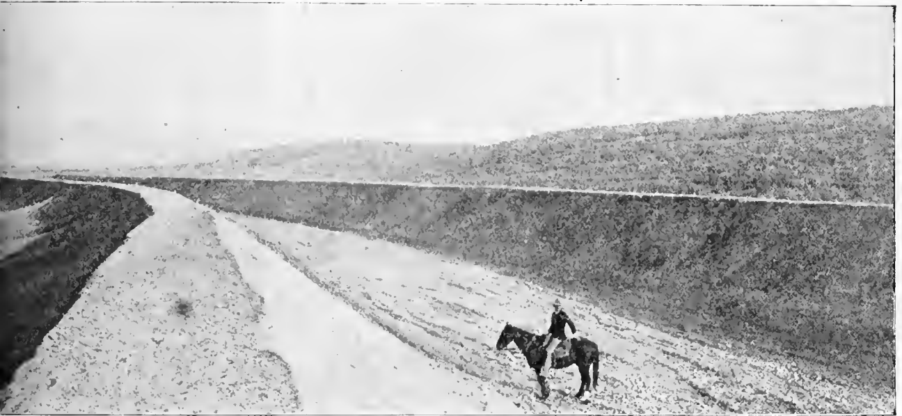
A NEW IRRIGATION DITCH, IDAHO.
