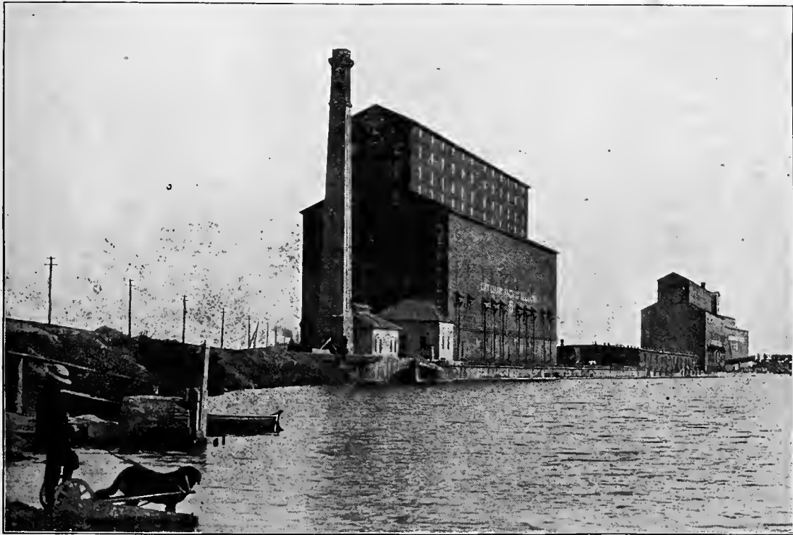
FORT WILLIAM ELEVATOR, CANADA.
