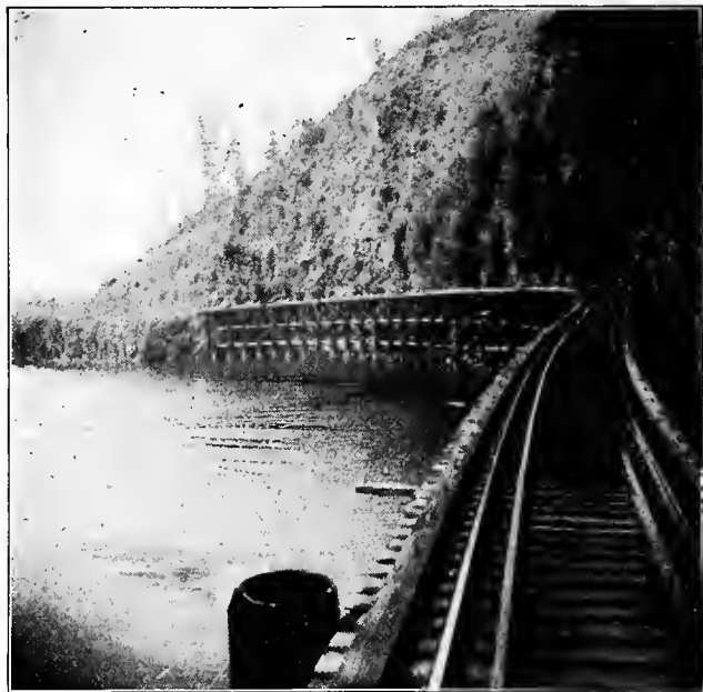
CREEPING ALONGSIDE THE MOUNTAIN ON THE TRESTLE.
