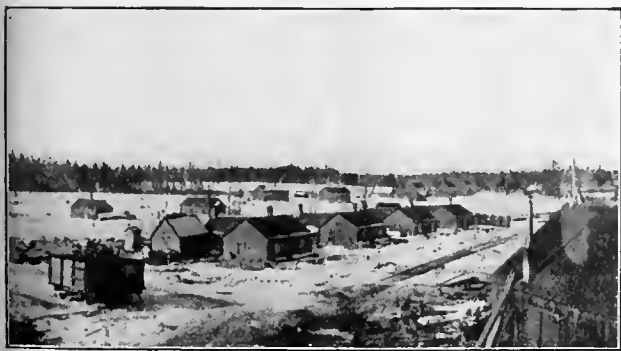
Viewing Skibo from the Mill.
