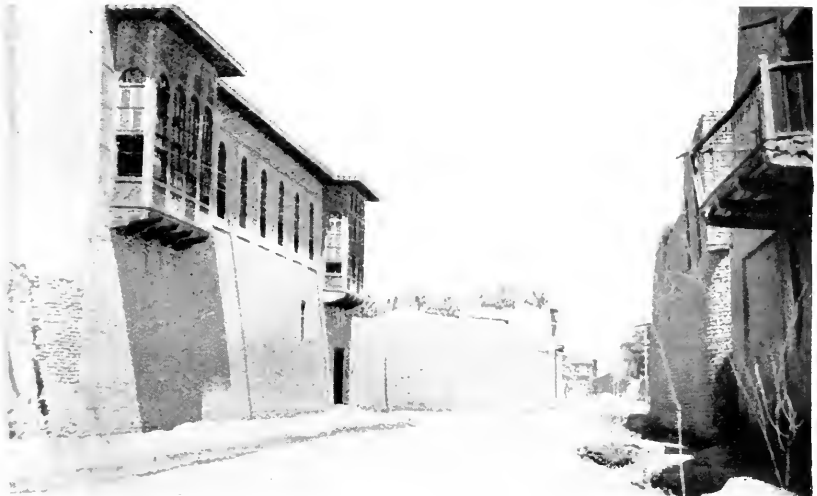
EXTERIOR OF THE A.P.O.'S BILLET (ON THE LEFT).
