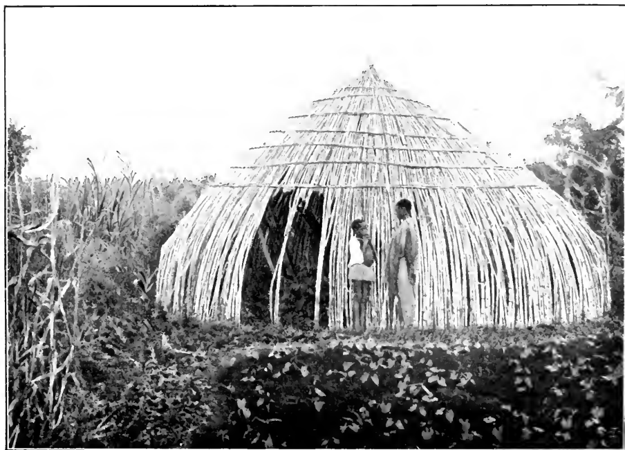
FRAMEWORK OF A WAHAIA HUT: BUKOBA DISTRICT
