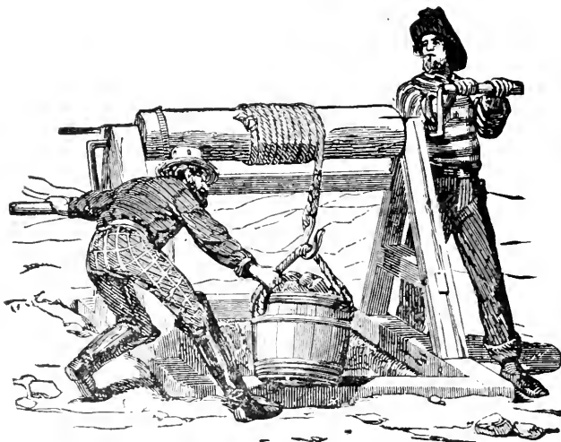
MINERS SINKING A SHAFT.
