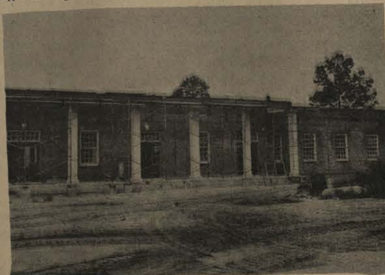
New budget cuts will halt campus construction.
