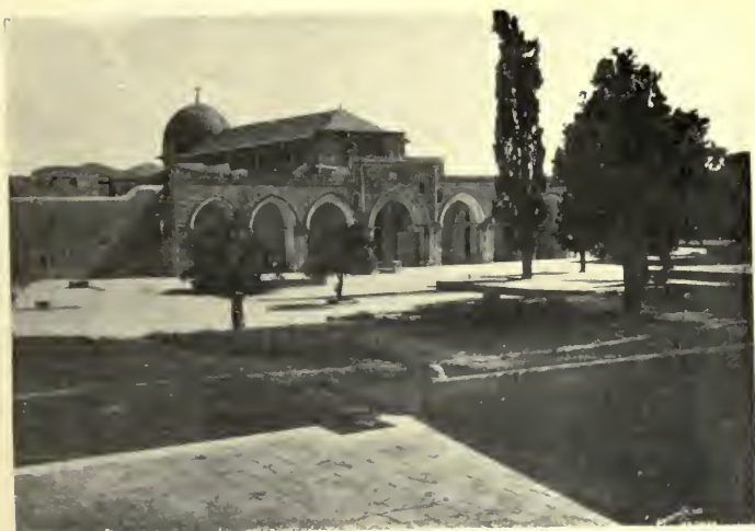
EL AKSA, "THE FURTHER MOSQUE."
