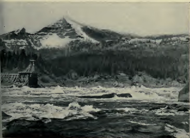
The north abutment of the Bridge of the Gods
