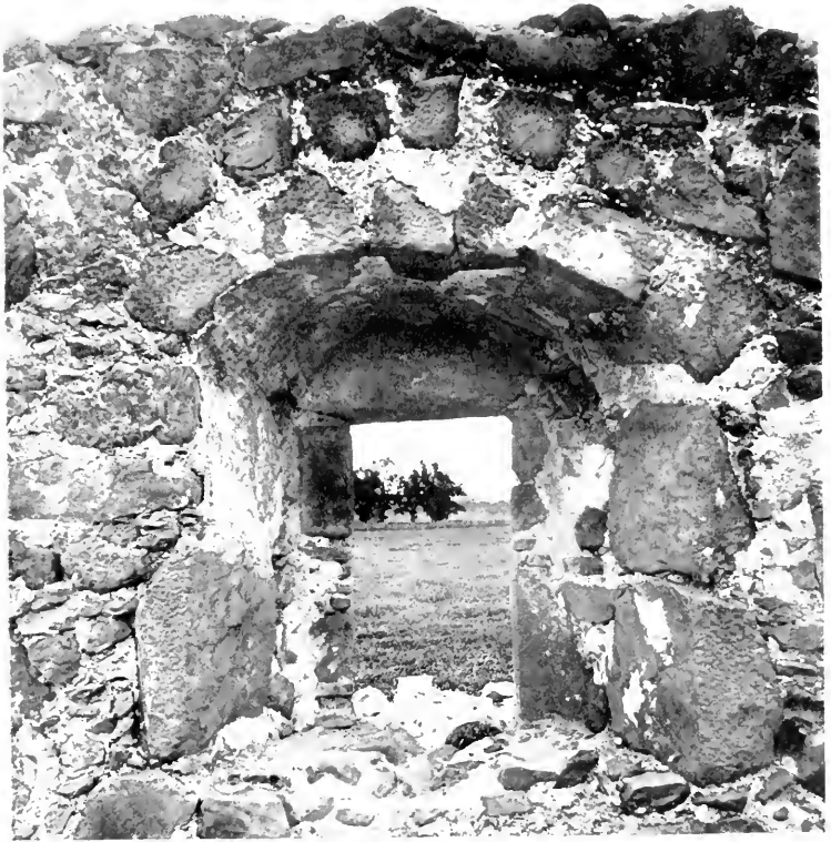
STONE ARCHED DOORWAY, SANTA MARGARITA CHAPEL.
