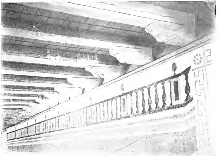
b. CORBELS AND RAFTERS OF SAN MIGUEL MISSION
