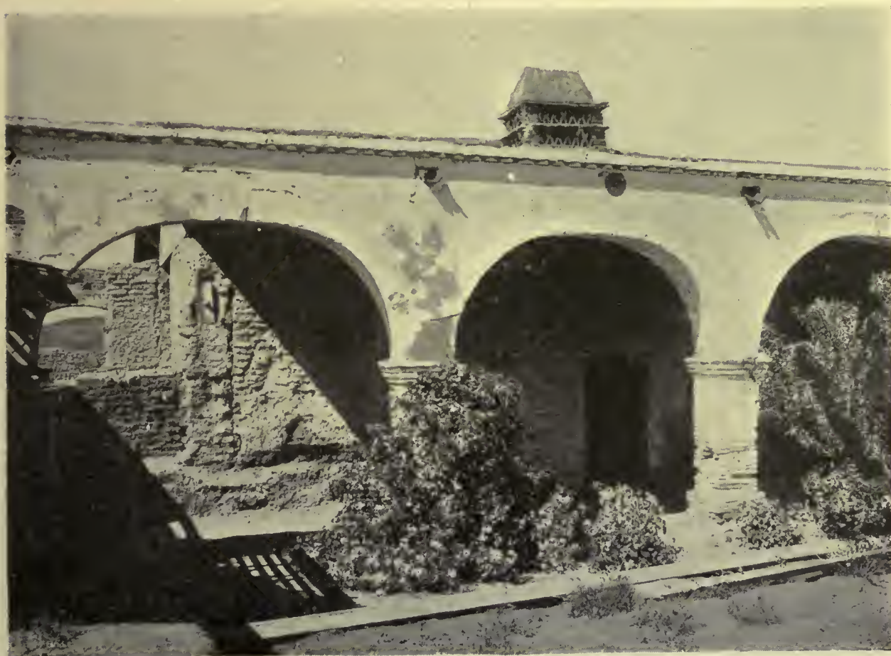
b. ELLIPTICAL ARCHES OF DIFFERING AXES, SAN JUAN CAPISTRANO
