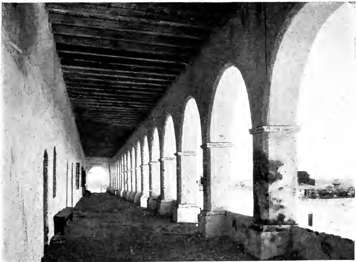
b. CORRIDORS AT SAN FERNANDO
