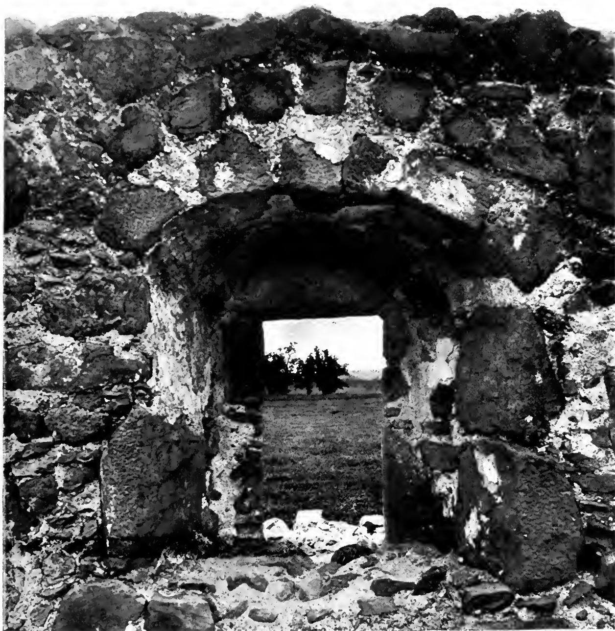
STONE ARCHED DOORWAY, SANTA MARGARITA CHAPEL
