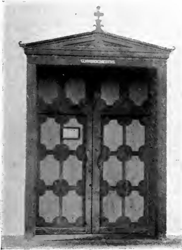
a. ENTRANCE DOORS, SAN MIGUEL
