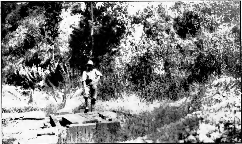
ENTRANCE TO INFILTRATION GALLERY AT SAN MANUEL
