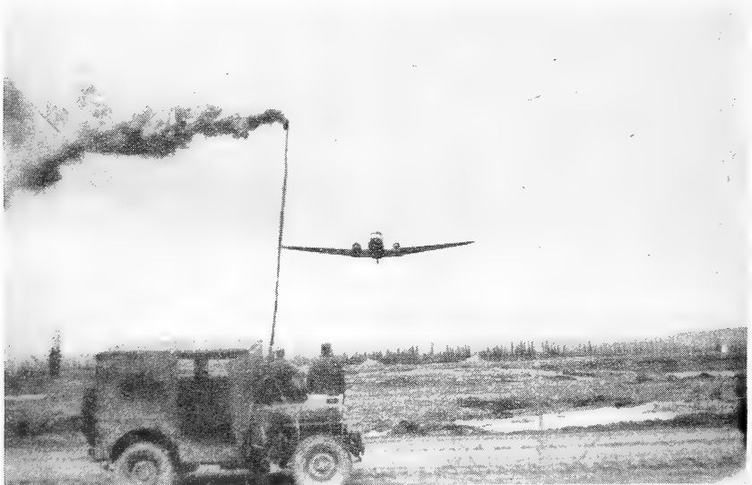
FIGURE 23.—Smoke grenade on a pole as marker for an airplane spray run.
