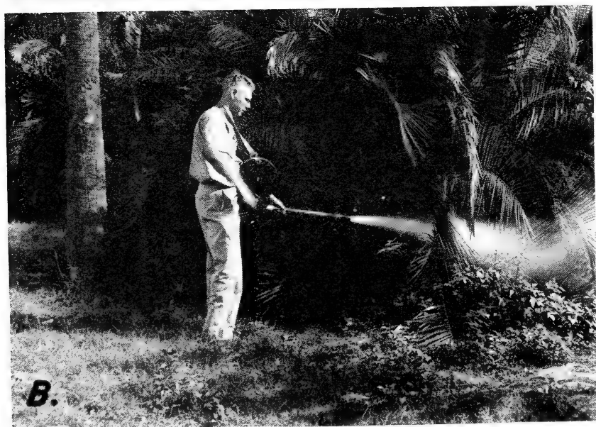
FIGURE 3.—Hand dusters: A, Plunger type; B, rotary type.
