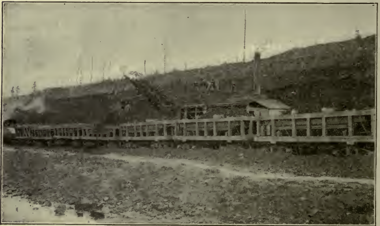
Shoveling ore from its native bed into cars.
