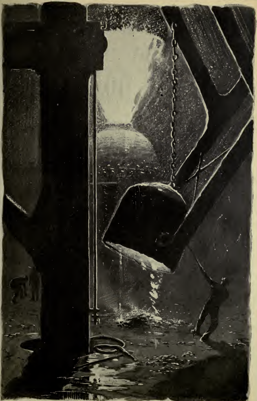
BESSEMER CONVERTER IN OPERATION
