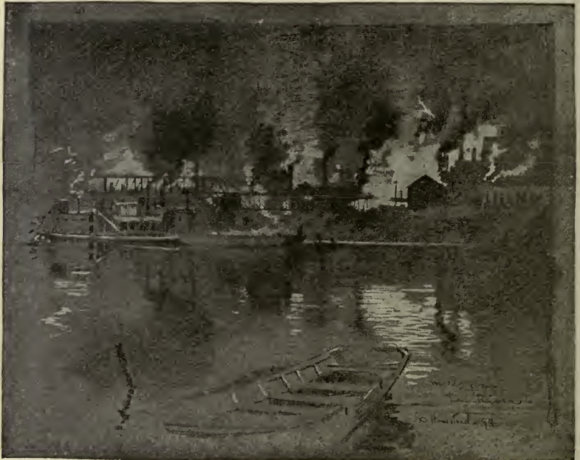
Steel works by night.
