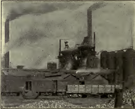
Lucy furnaces, showing hot-blast stoves.
