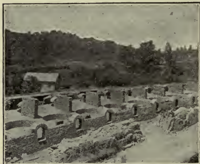
Coke-ovens under construction.
