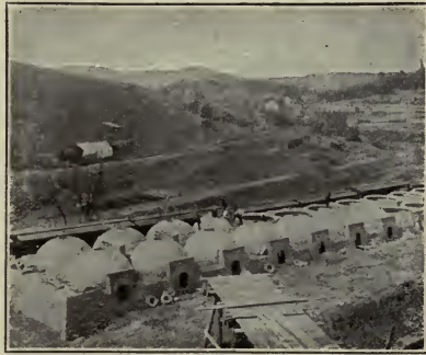
Coke-ovens under construction.
