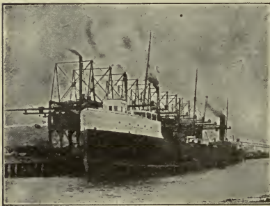
Ore-discharging machines at Conneaut.
