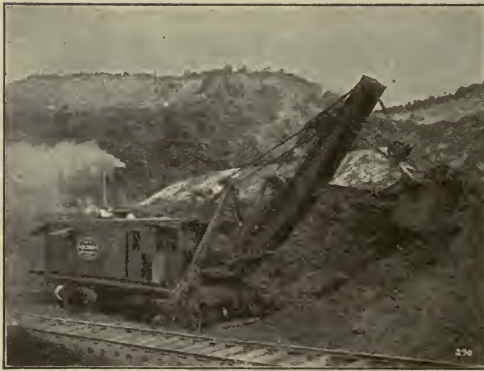
A BUCYRUS SHOVEL AT WORK. "Five cents a ton for labor."
