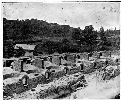
Coke-ovens under construction.
