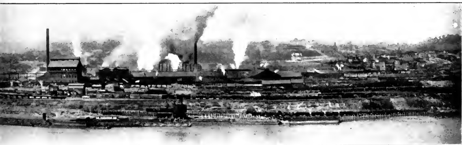
WORKS, DUQUESNE, PA.
