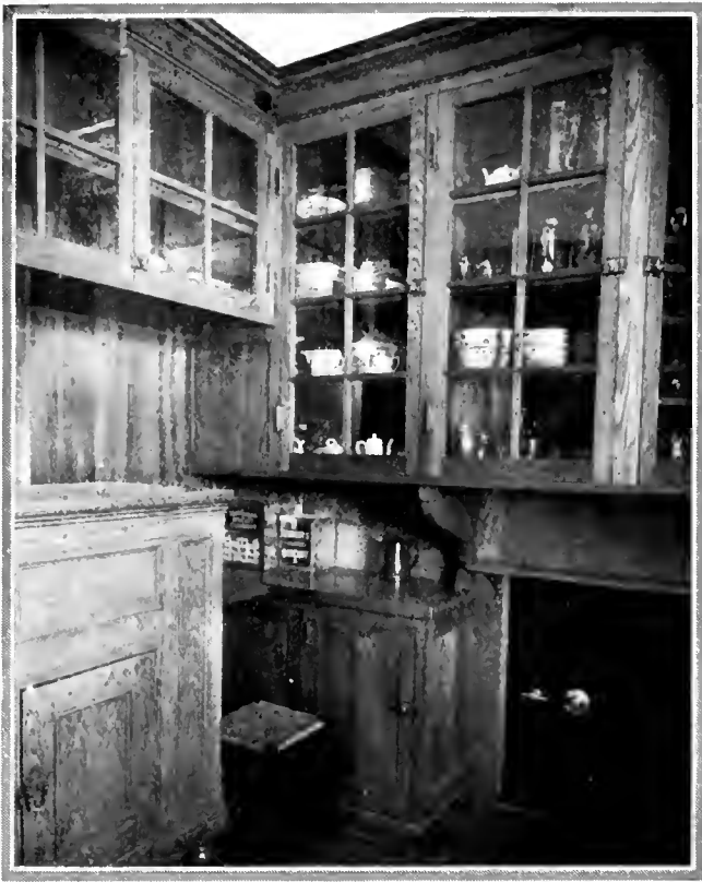
A PANTRY presents endless opportunities for convenient devices. This one has a safe for the nightly locking up of the silver in constant use and for the storage of less-used pieces. The shelving is well thought out, and a low stool provides a means of reaching the topmost dishes. Every available space is used for shelf and cupboard room.
