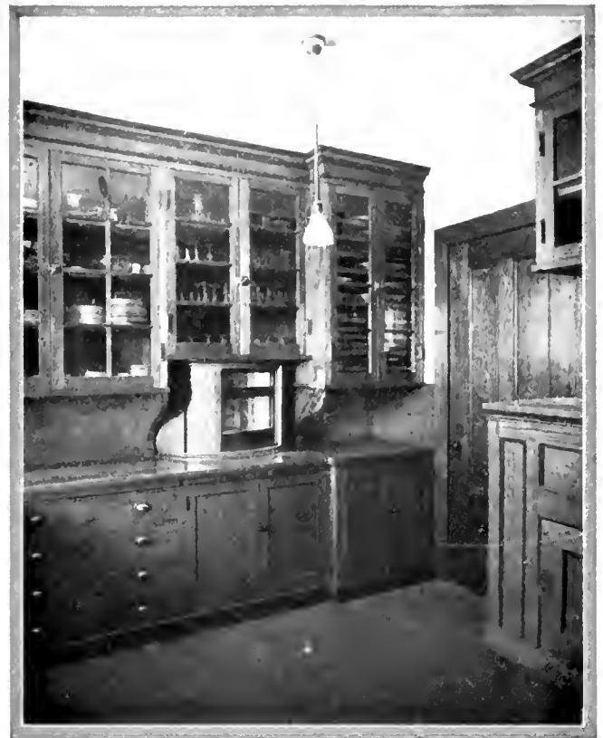
A SOLUTION of the problem of keeping kitchen odors out of the rooms is offered by the installation of a turnstile slide between kitchen and pantry. If the expense of this turnstile is an item to be considered, the usual wooden slide may be fitted with a large glass panel, which acts as a bar to odors, although not, of course, so effectively as the turnstile.
