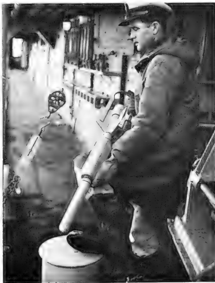
Figure L-14. A spring scale dynamometer.
