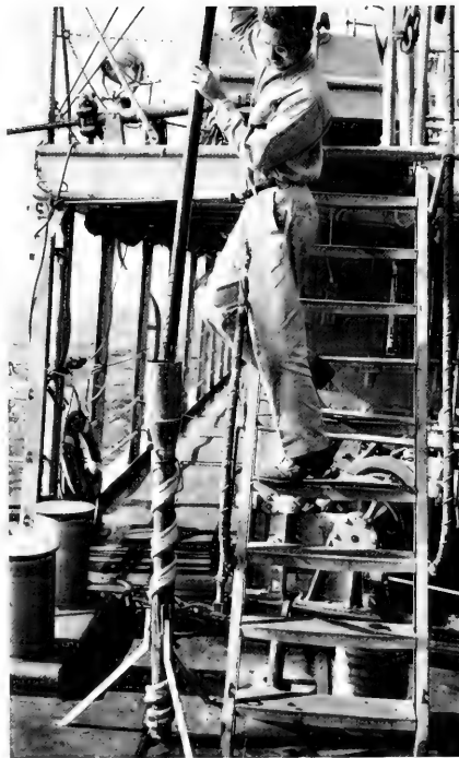
Figure L-16. Applying wax to a plastic liner.
