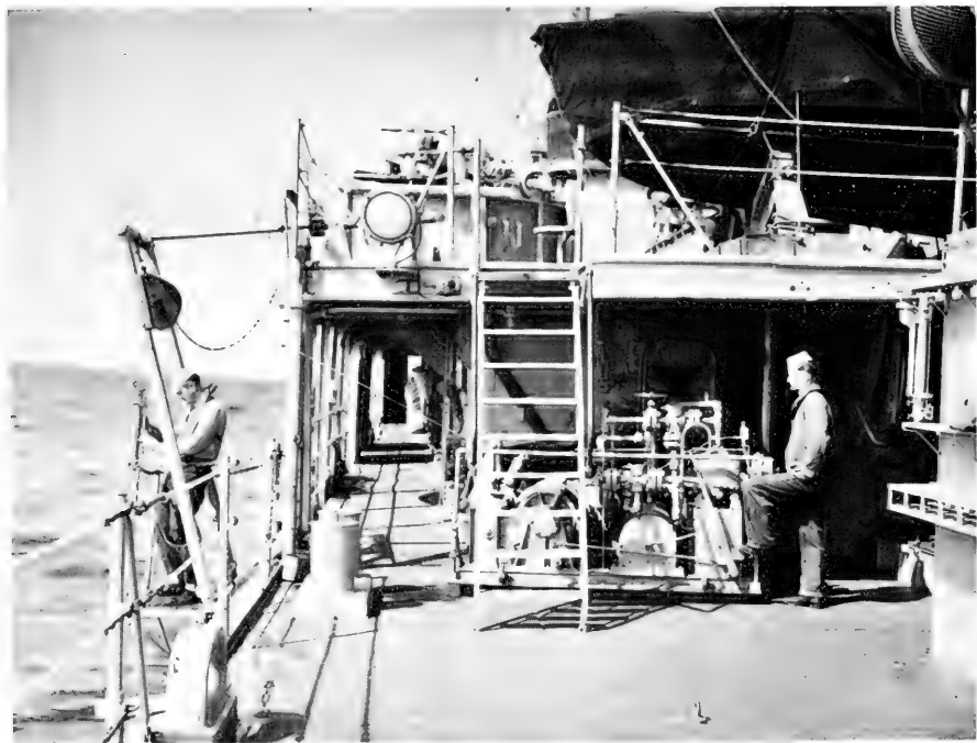
Figure 1-1. View of A-frame, platform, and oceanographic winch.
