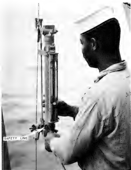
Figure E-4. Nansen bottle being placed on wire.
