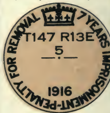
Fig. 19. \frac{1}{4} sec. cor. on South By. 5-147-13 E. Quarter sec. cor. north of correction line.
