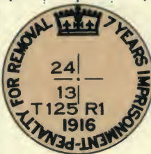
Fig. 15. N.E. cor. 13-125-1 Sec. cor. on initial meridian
