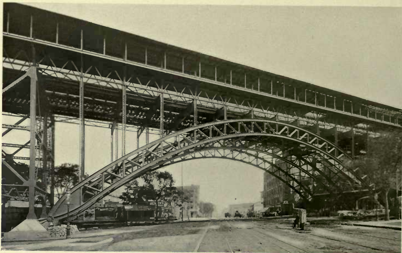
COMPLETED ARCH AT MANHATTAN STREET
