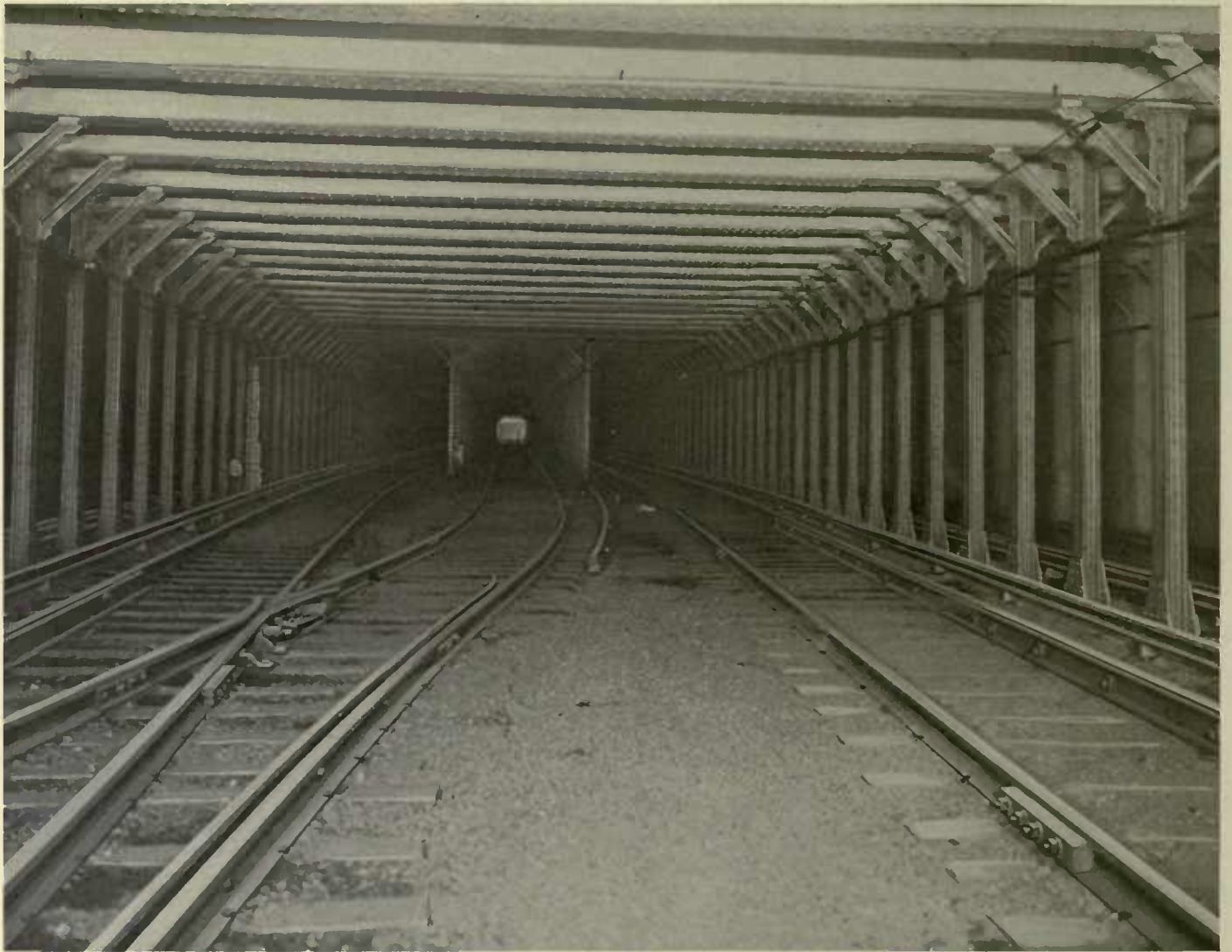
FOUR-TRACK SUBWAY — SHOWING CROSS-OVER SOUTH OF 18TH STREET STATION
