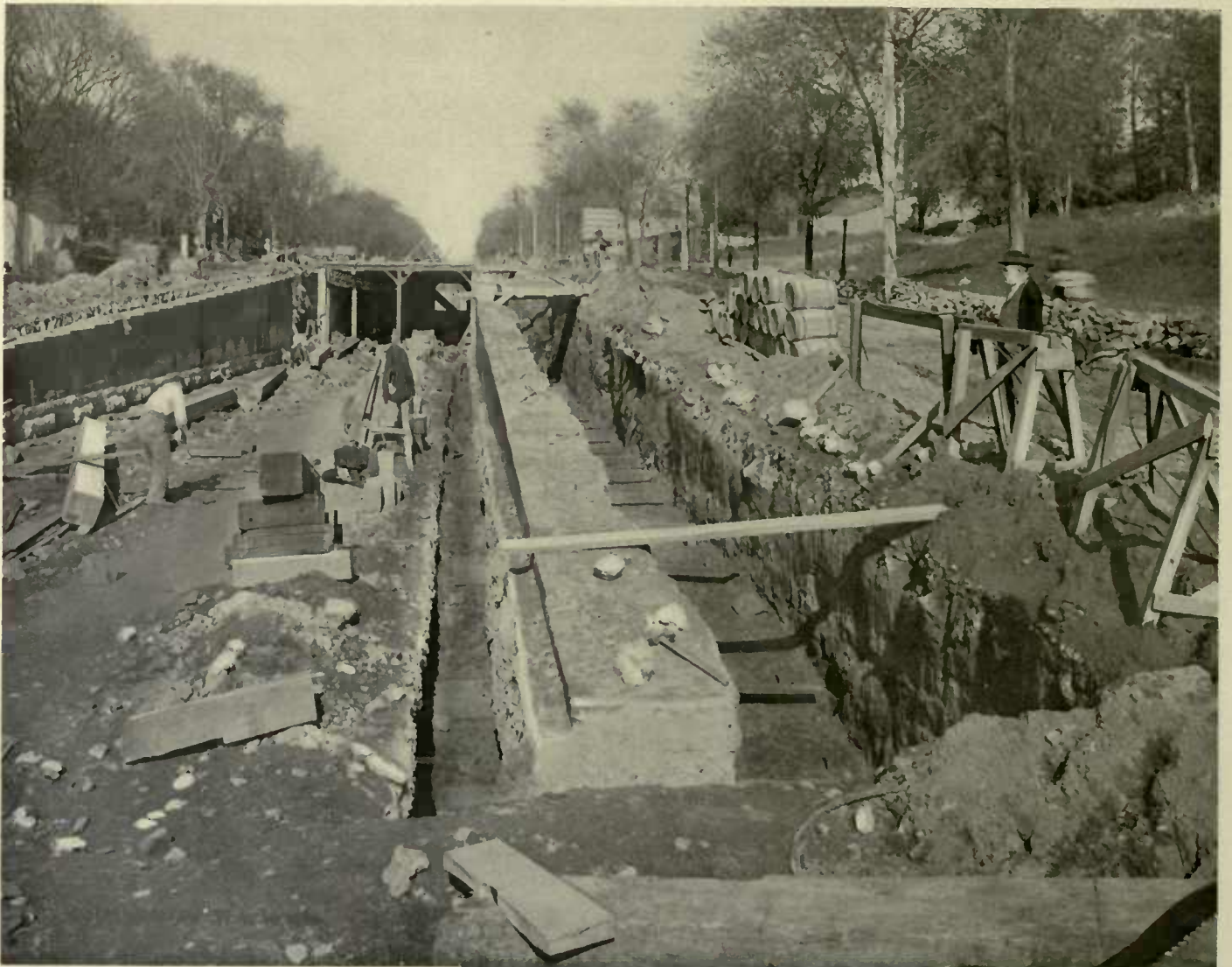
MOVING BRICK AND CONCRETE RETAINING WALL TO MAKE ROOM FOR THIRD TRACK—BROADWAY AND 134TH STREET
