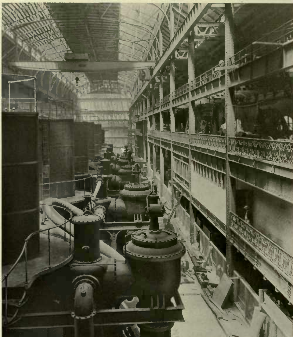
OPERATING ROOM SHOWING CONDENSERS — POWER HOUSE
