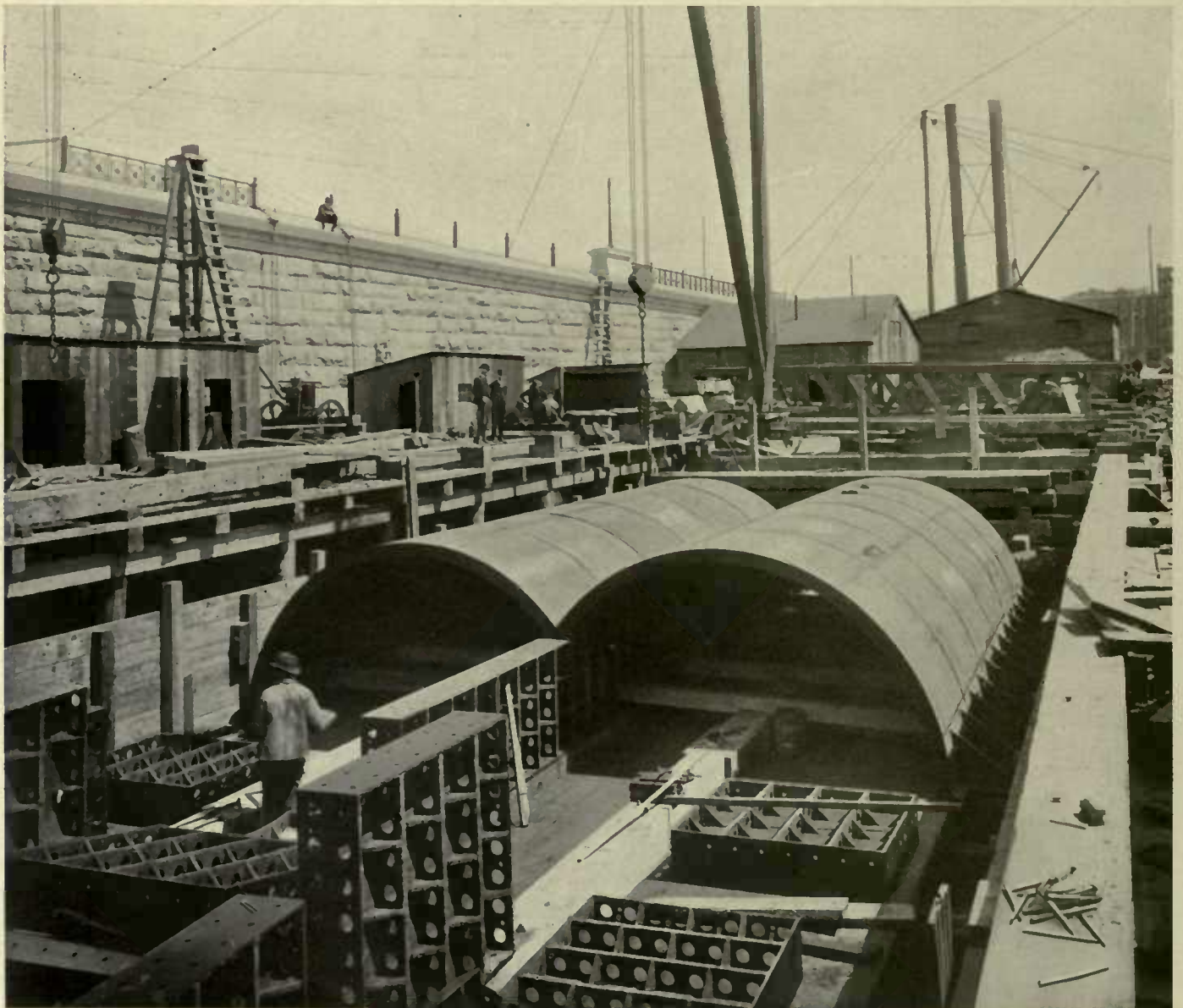
ASSEMBLING IRON WORK ON PONTOON—HARLEM RIVER TUNNEL
