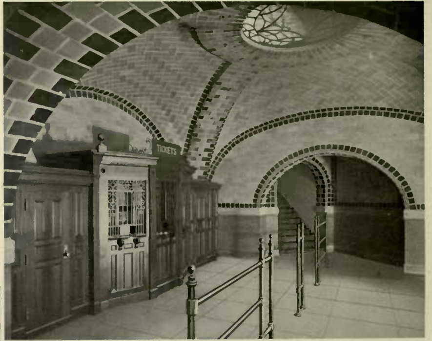
CITY HALL STATION
