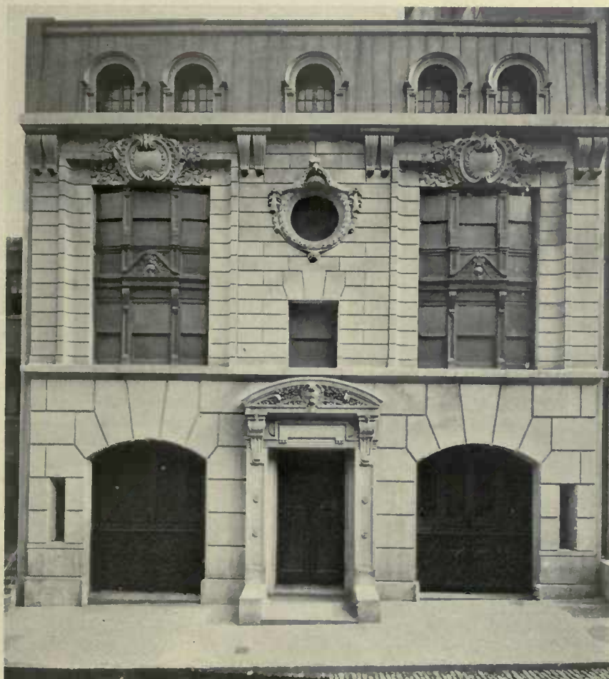
EXTERIOR OF SUB-STATION NO. 11
