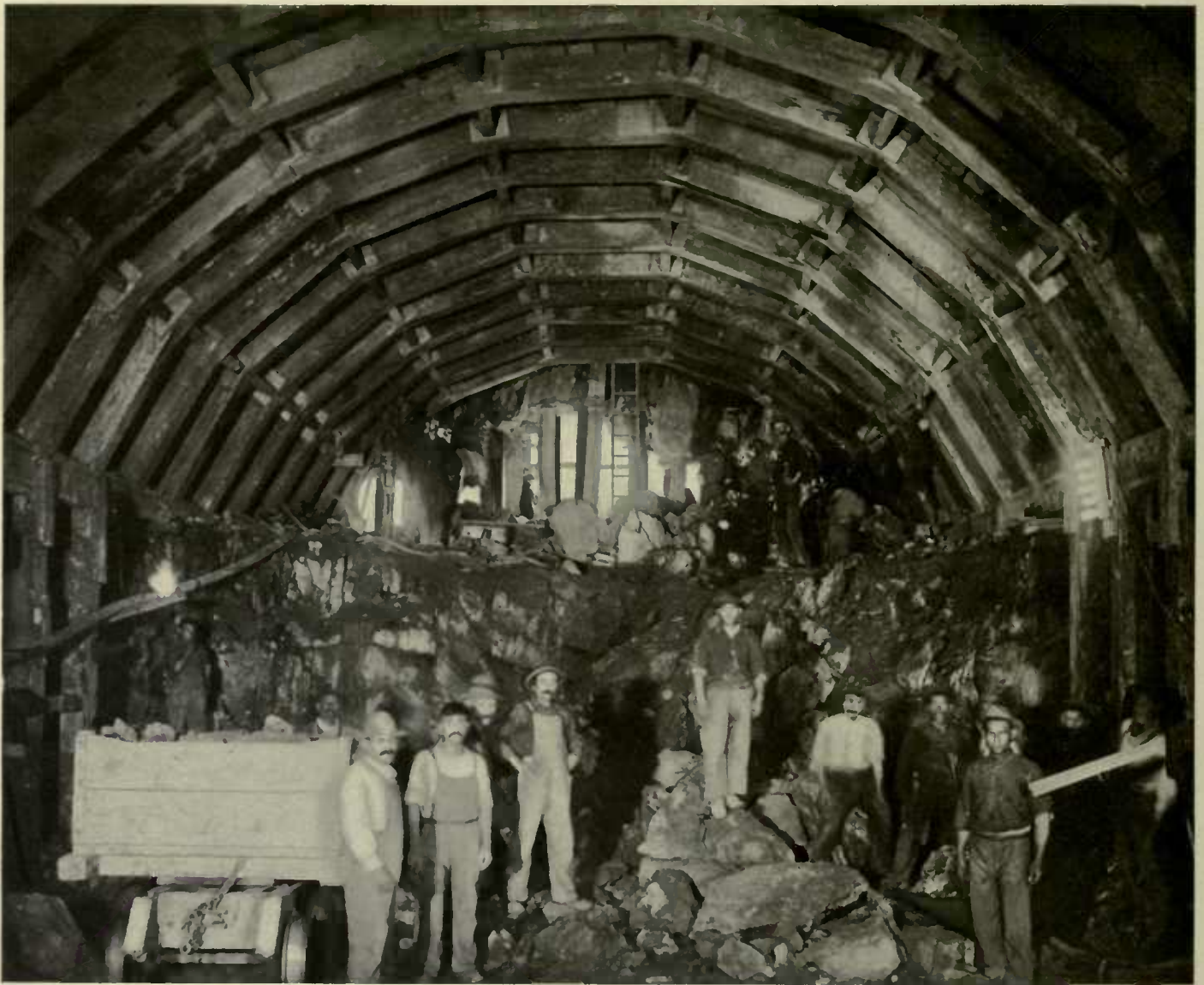
CONSTRUCTION OF FORT GEORGE TUNNEL
