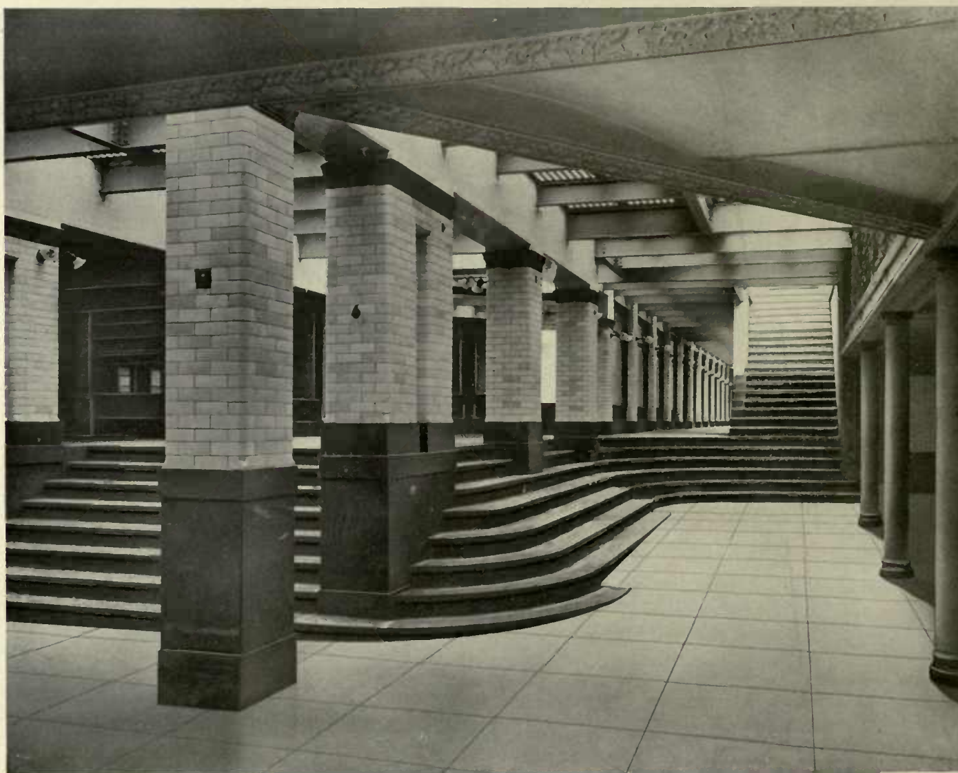
WEST SIDE OF 23D STREET STATION
