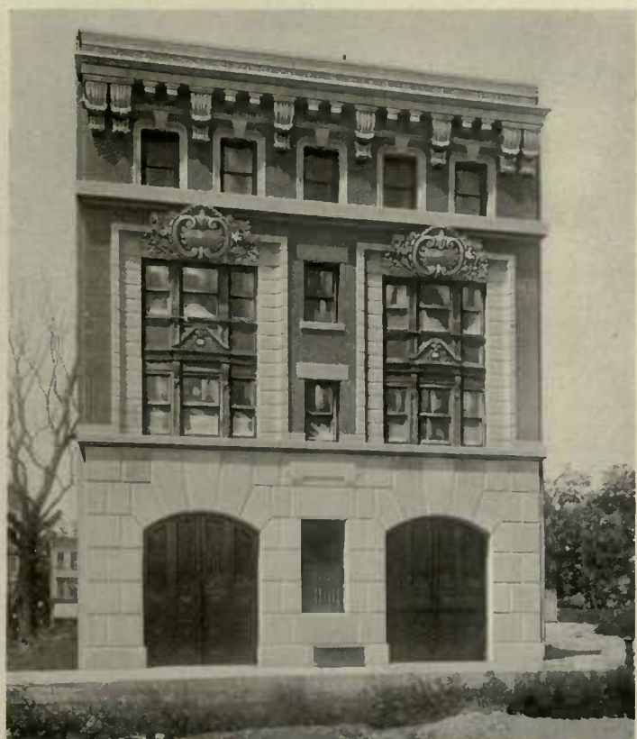
EXTERIOR OF SUB-STATION NO. 18
