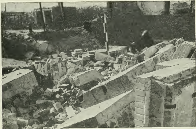
FIGURE 4.— Upper photo: Building with load-bearing walls, 5,200 feet from ground zero. Load-bearing wall away from the blast collapsed. Lower photo: Interior of same building, showing damage from blast and fire.
