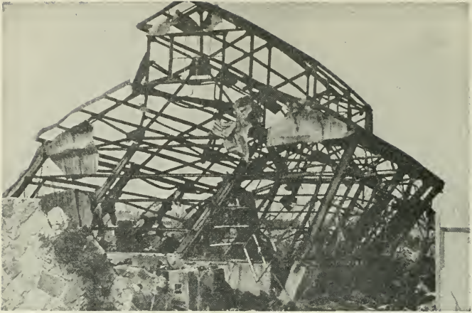
FIGURE 3.—Light, steel-frame industrial building, 1,800 feet from ground zero (ground point directly beneath the explosion). Corrugated iron roof and wall sheathing were stripped by the blast, and the combustible contents destroyed by fire.
