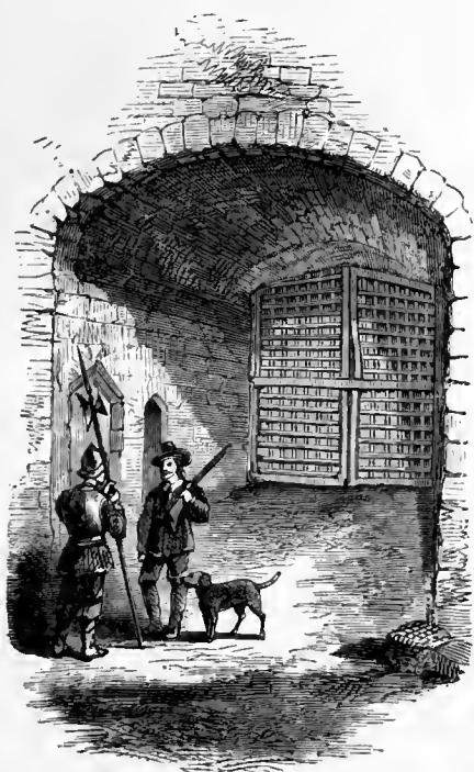
GATEWAY UNDER THE EAGLE TOWER.
