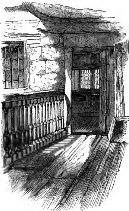
GALLERY ACROSS SMALL YARD.
