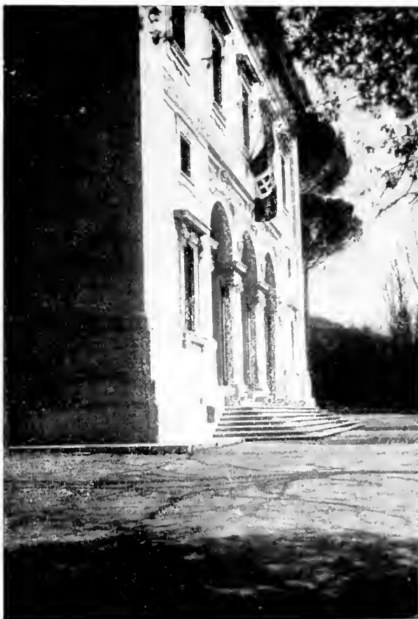
DETAIL OF THE FAÇADE.
