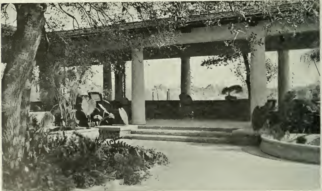
COURT ON EAST SIDE OF MR. GILBERT E. PERKINS' HOUSE AT PASADENA, CALIFORNIA
