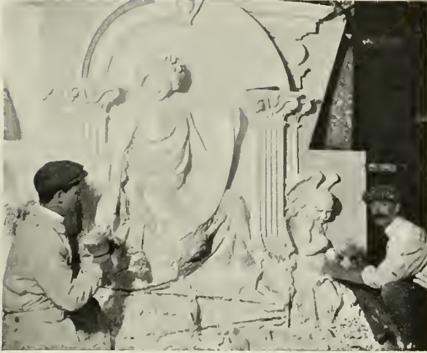
FIG. 4.—CHIPPING THE WASTE MOULD
