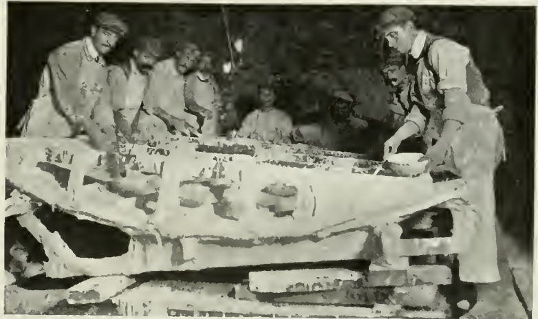
FIG. 6.—MAKING CASE FOR GELATINE MOULD
