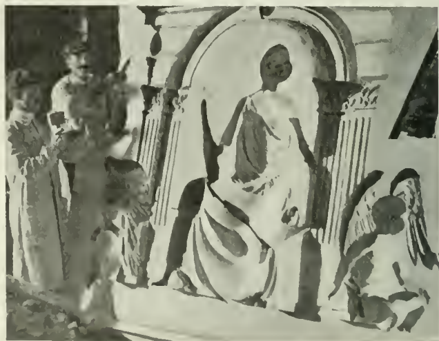
FIG. 3.—THE WASTE MOULD
