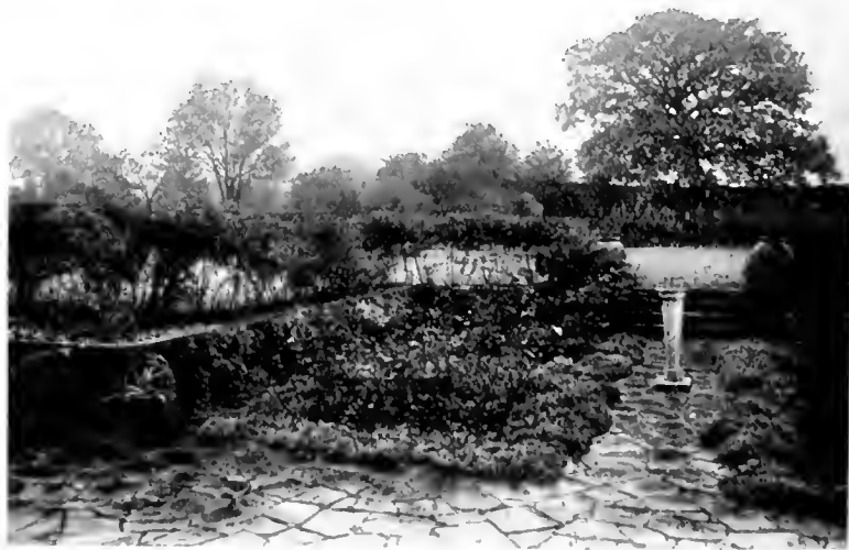
BERRYDOWN COURT, OVERTON: THE ROSE GARDEN EDWIN L. LUTYENS, ARCHITECT
