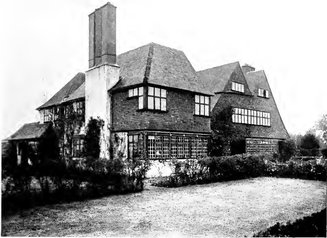
BERRYDOWN COURT, OVERTON: SOUTH FRONT
