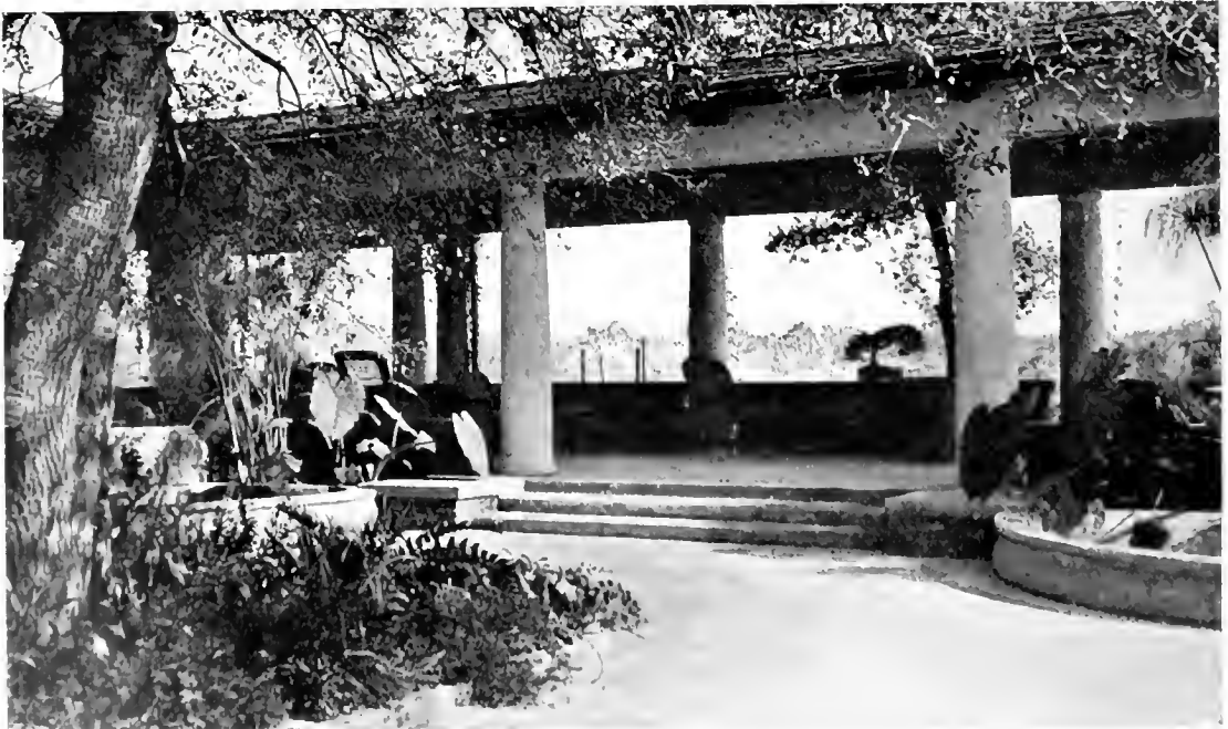
COURT ON EAST SIDE OF MR. GILBERT E. PERKINS' HOUSE AT PASADENA, CALIFORNIA
