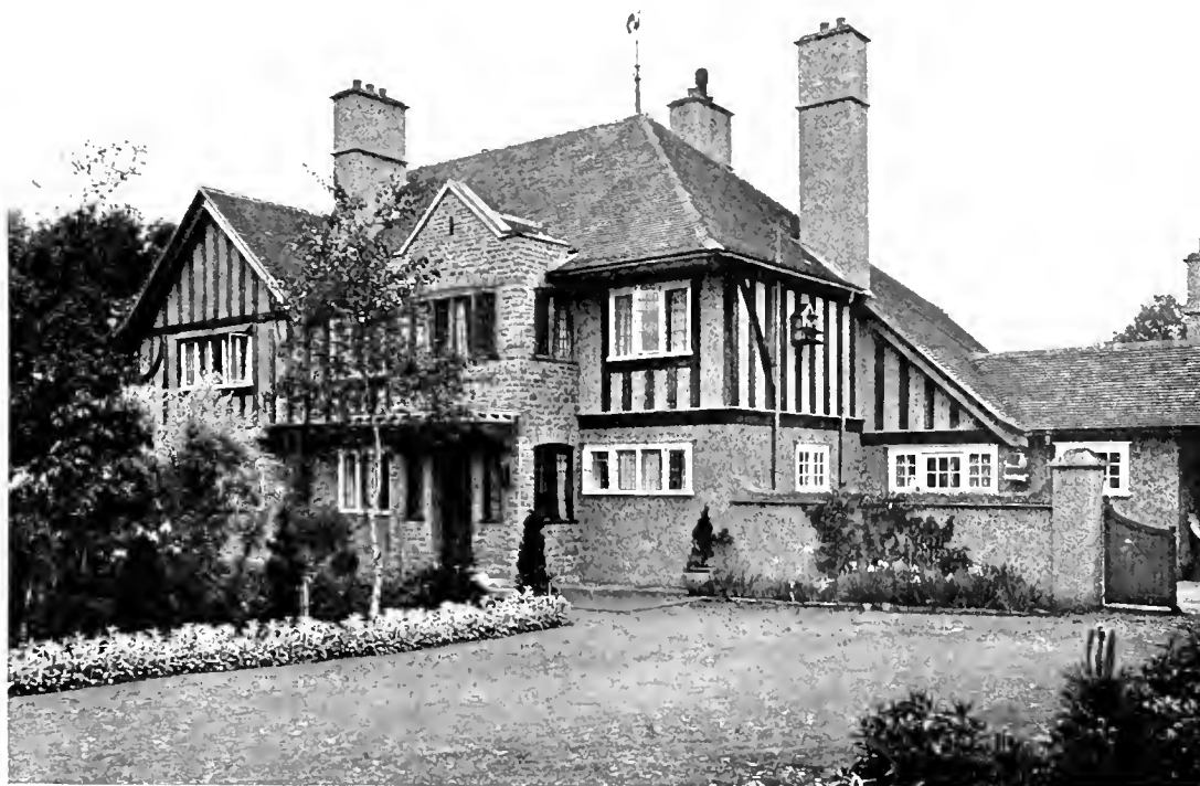
GATE HOUSE, SHACKLEFORD COMMON: GARDEN VIEW
