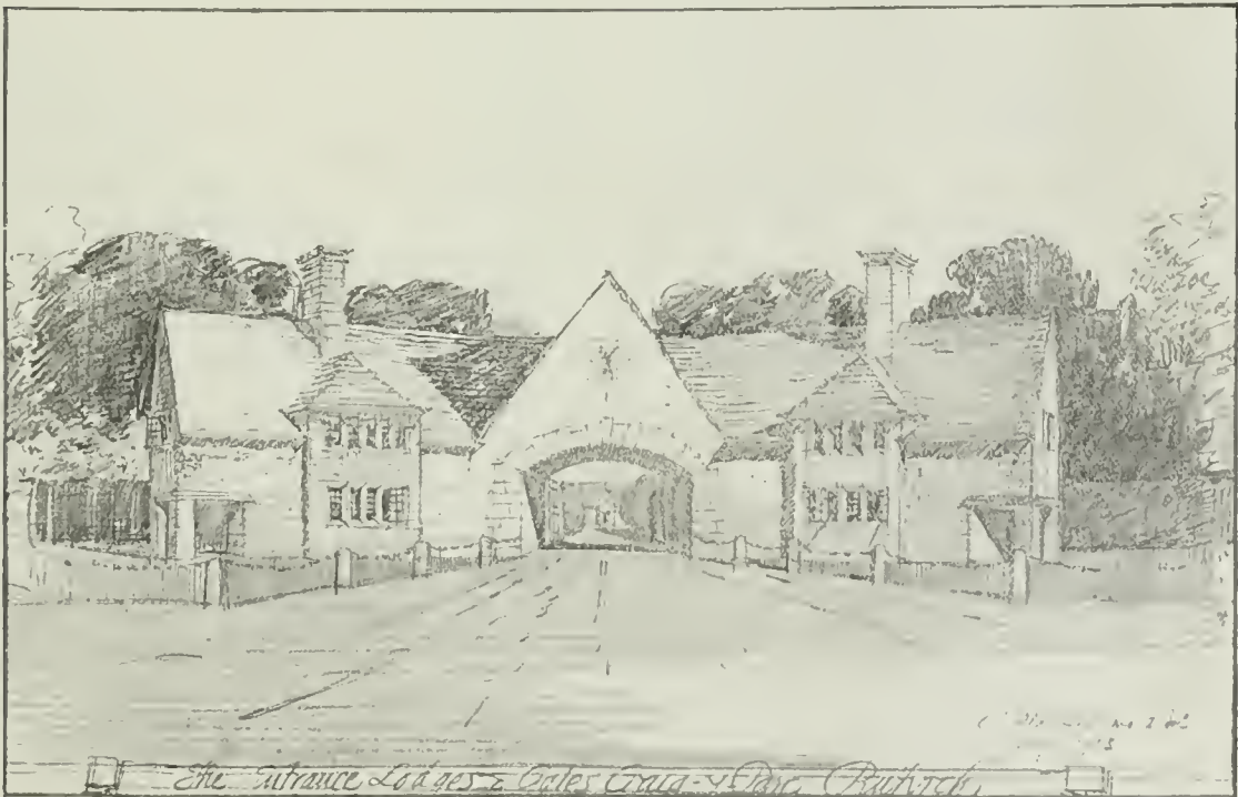
CRAIG-Y-PARC, NEAR CARDIFF: ENTRANCE LODGES
