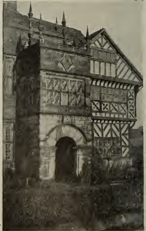
HALL-I' TH'-WOOD, BOLTON: SOUTH PORCH
