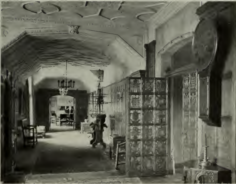
GALLERY SHOWING THE STEEL GRILLES. DINING-ROOM BEYOND THE SCREEN
