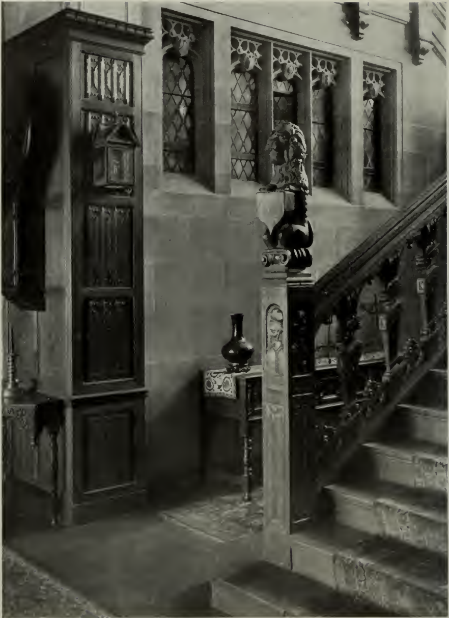
A CORNER OF THE MAIN STAIRWAY
