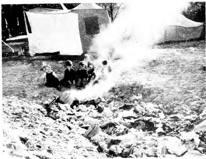
Defense construction workers' children playing around garbage and rubbish heap in the rear of their tent homes near Camp Livingston, La. December 1940
