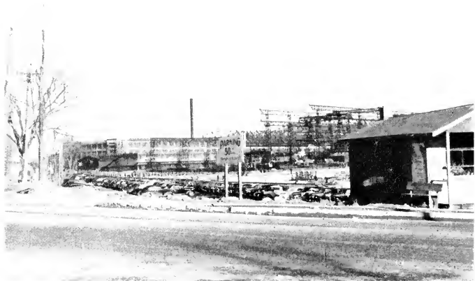
Parking lot adjoining Quincy, Mass., shipyards. Cars parked here bear tags from many States.
