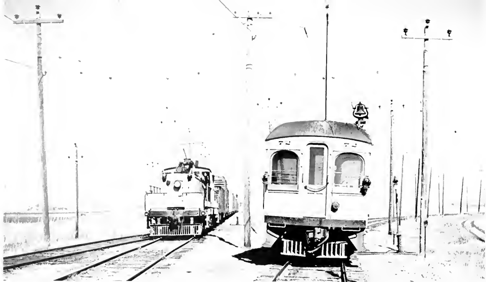
A four-truck locomotive that once wheeled Oregon Electric tonnage through the Willamette Valley had backed its Fort Dodge Line train into the Rockwell City branch at Hope to clear a northbound car. WILLIAM D. MIDDLETON.
