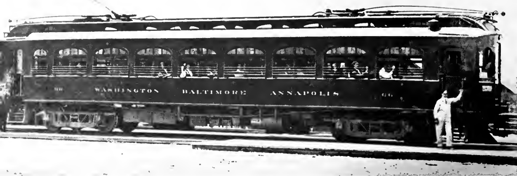
The impressive dimensions of the W&B&A's Niles "Electric Pullmans" are evident in a broadside study. The big cars regularly clocked 66-mile-per-hour average speeds once they got out of town. LEROY O. KING COLLECTION.
