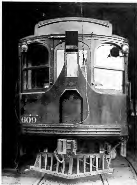
A less successful interurban experiment was this bizarre device applied to the front end of a Buffalo & Lake Erie Traction car which was designed to utilize heat from the headlight to defrost the front windows. STEPHEN D. MAGUIRE COLLECTION.
