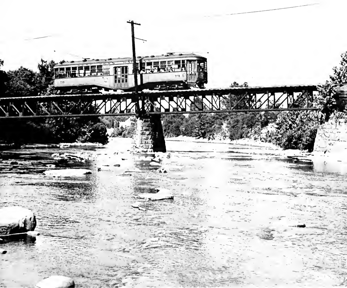
A few shirt-sleeved passengers gazed momentarily upon the waters of Loyalbanna Creek as car 711 sped across a bridge on the Latrobe line in 1952. JOHN STERN.
