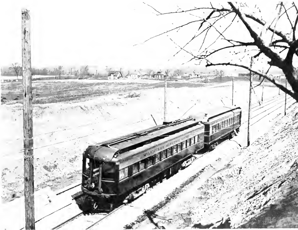
Work was still under way on the Milwaukee Electric's new rapid-transit route to West Junction when this rebuilt motor car and trailer came out of the shops for a 1926 inspection trip. Car 1111 was soon nicknamed the Four Aces by crews. STATE HISTORICAL SOCIETY OF WISCONSIN.
