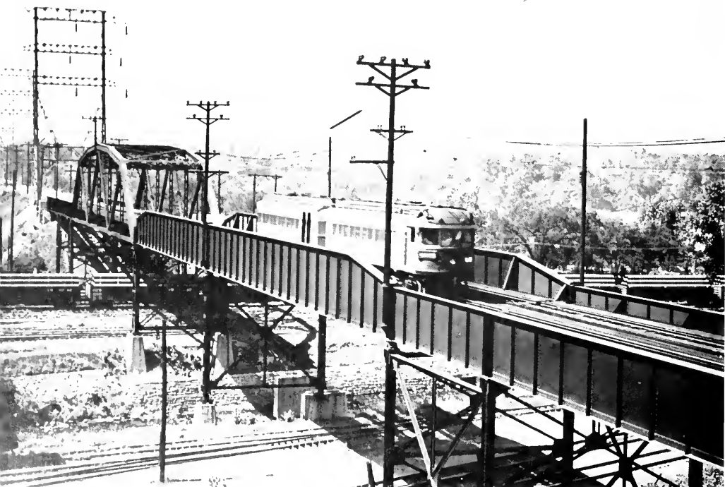
One of the articulated "duplex" units rebuilt by T.M.E.R.&L. shops from conventional equipment in 1929 crossed the substantial steel structure that carried the rapid-transit route over the Menomonee River and the Milwaukee Road main line. WILLIAM D. MIDDLETON.
