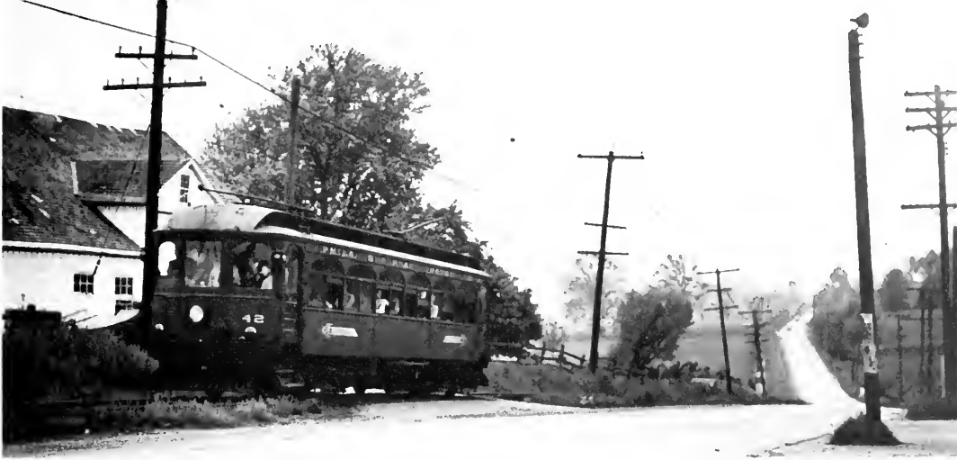
The roadside development often characteristic of interurbans is illustrated here by the West Chester line of the Philadelphia Suburban Transportation Company. The 1914 Jewett interurban shown was junked a few months after this 1949 photograph was made, but the line itself continued to operate for another five years with streamlined equipment. CHARLES A. BROWN.
