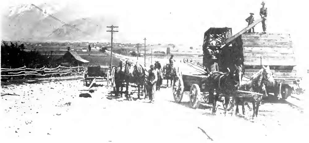
Motorized construction equipment was still in the future even during the last years of interurban development, when the Salt Lake & Utah constructed its line into Payson, Utah, on the eve of World War I. FRED FELLOW COLLECTION.
