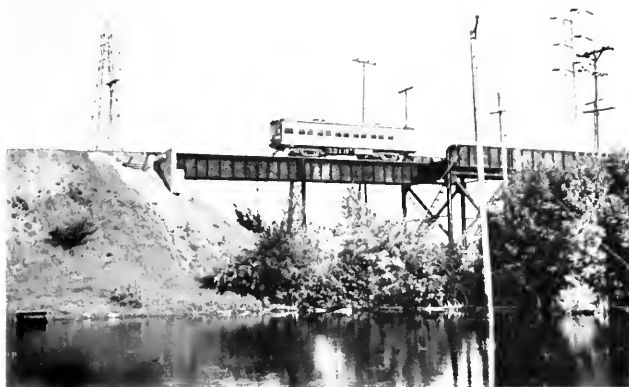
Inbound from Hales Corners in 1949, a Milwaukee Electric interurban crossed over the Chicago & North Western at West Junction on a bridge that was clearly constructed to accommodate future multiple track. The structure was part of a mile-long cutoff completed in 1927 which afforded Burlington and East Troy interurbans access to the new rapid-transit entry to Milwaukee, cutting 23 minutes from previous running times via city streets. WILLIAM D. MIDDLETON.
