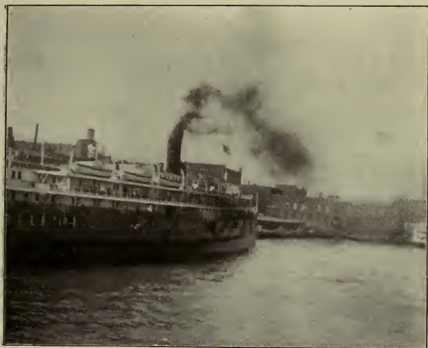
THE WATERSIDE, CLEVELAND.
