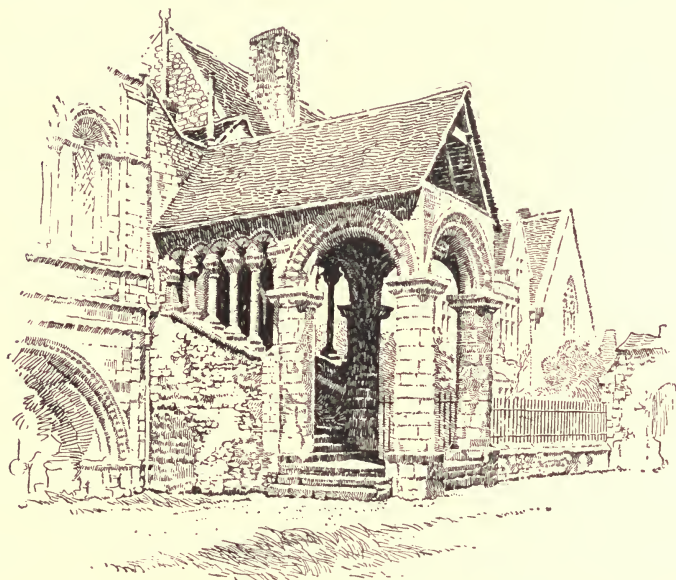
NORMAN STAIR, CANTERBURY
