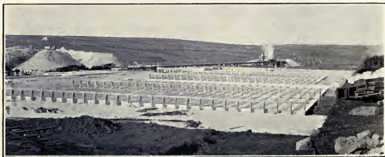
Mica drags at Stannon Works of North Cornwall China Clay Co., Ltd.
