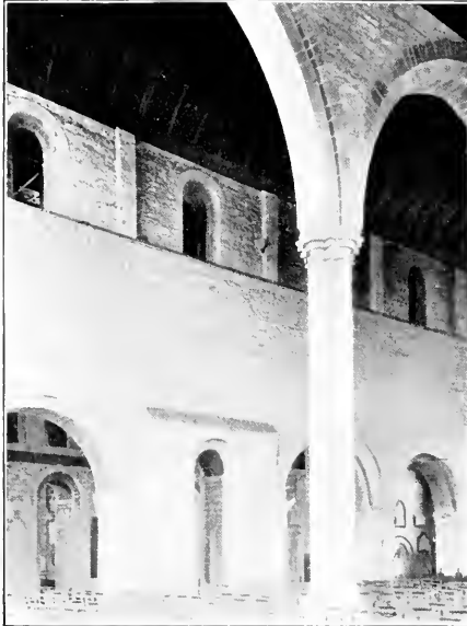
F. B. Leominster: Exterior of Norman Nave from S.W.
