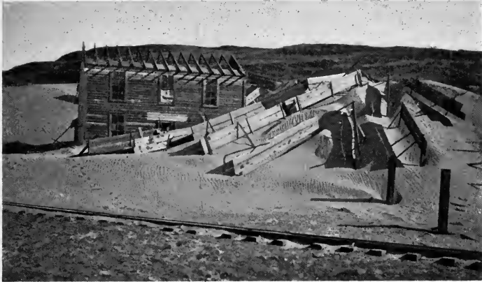
FIG. 84.—The last house in Biggs, Ore., a village overwhelmed by dunes. Attempts to hold the sand back by fences were unsuccessful.
