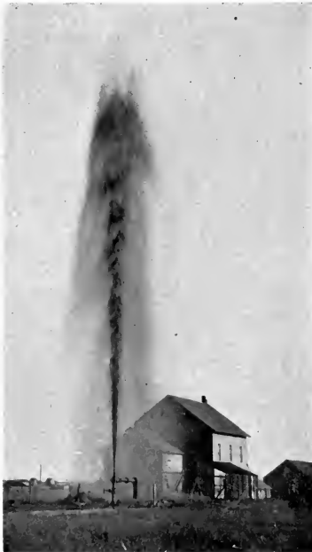
FIG. 76.—Artesian well at Woonsocket, S. Dak. When photographed the jet was 97 feet high.
