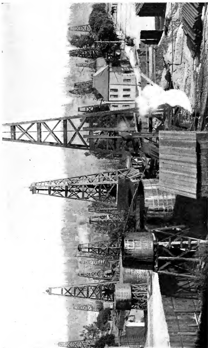
FIG. 248.—Oil-wells in Los Angeles, Cal. Each well has a tall "derrick," used in handling the drilling machinery.
