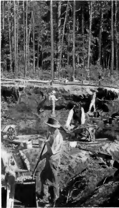
FIG. 135.—Placer mining in North Carolina. The gold is separated from the contained earth by means of a swift current of water.
