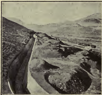
FIG. 221.—Irrigation canal into which water is diverted for distant ranches.
