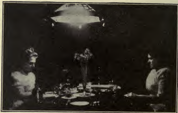
FIG. 118. — A poorly arranged light in a dining room.
