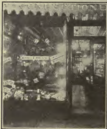
FIG. 121. — A well-lighted display at the left. The lamps are concealed. A poorly lighted window at the right. The bright unconcealed lamps produce a glare.
