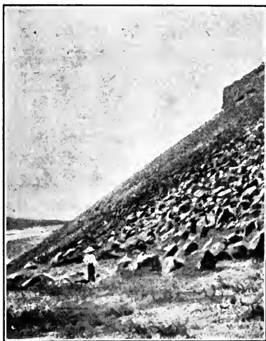
FIG. 25. — The destruction caused by freezing water.
