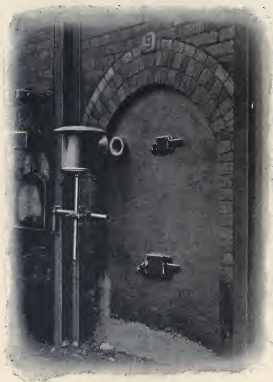
FIG. 34.—Féry Radiation Pyrometer, for taking Temperature of Pottery Kiln.
