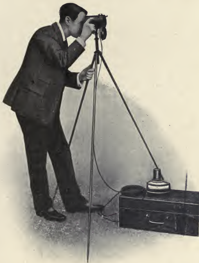
FIG. 35.—Sighting a Féry Radiation Pyrometer.
